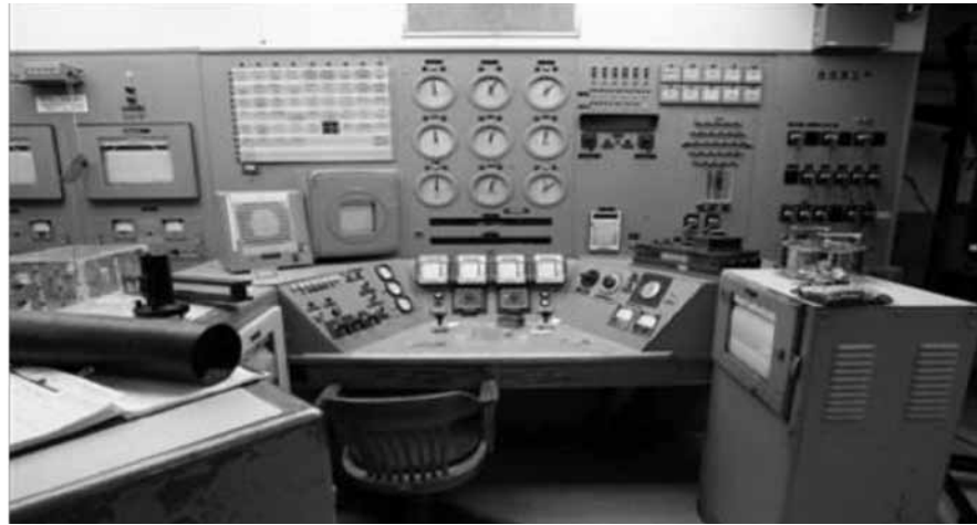
The control room within B-Reactor, where a push of a single button could have raised the rate of plutonium production or shut it down completely in case of emergency.
